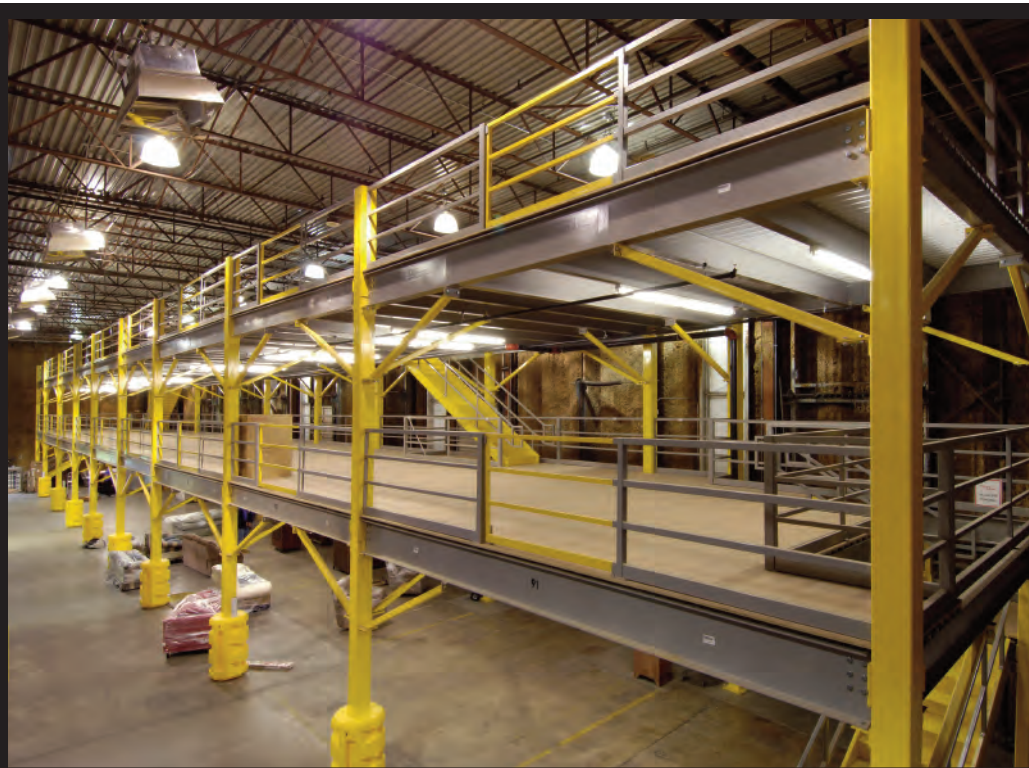
Excel Storage Products designed this 2-level mezzanine for a furniture warehouse, which includes stairs, telescoping gates and extra heavy-duty column protection.
