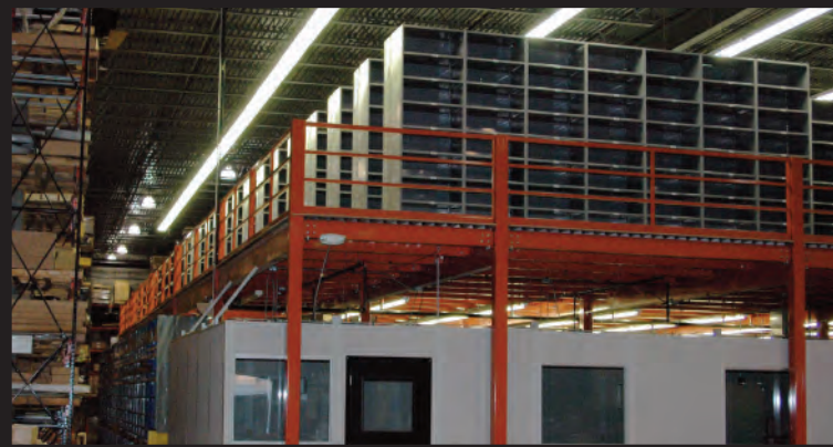
Top: Space is optimized by constructing a mezzanine in this new facility
